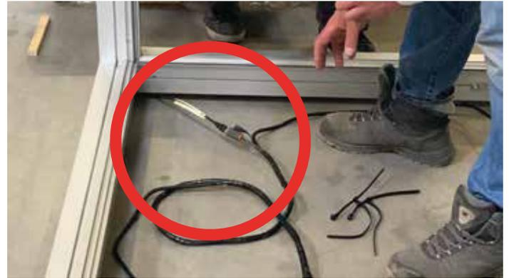
3.4 Connect USB Cables to the cables in the frame
